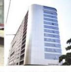
glass and also panel elevation. At some places, the structure took curved shape as per elevation. False structure was made to take exact curved shape made up of lighter sections of RHS & SHS which were connected to main PEB members which are segmented to take the shape
